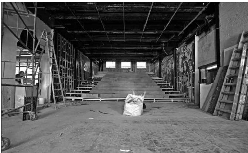
Yaron Yerushalmi's theater is undergoing renovation
