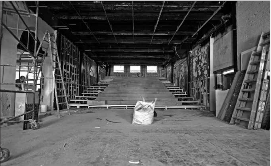
Yaron Yerushalmi's theater is undergoing renovation
